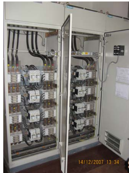
Fig. 7: The PFC system
